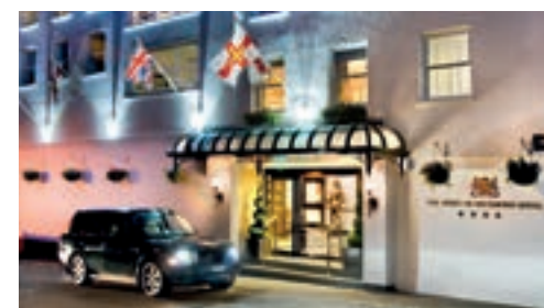
Pictures top to bottom: The spa at the Royal Yacht Hotel; Duke of Richmond Hotel.
